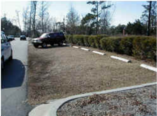
Parking Lot with Porous Surface
